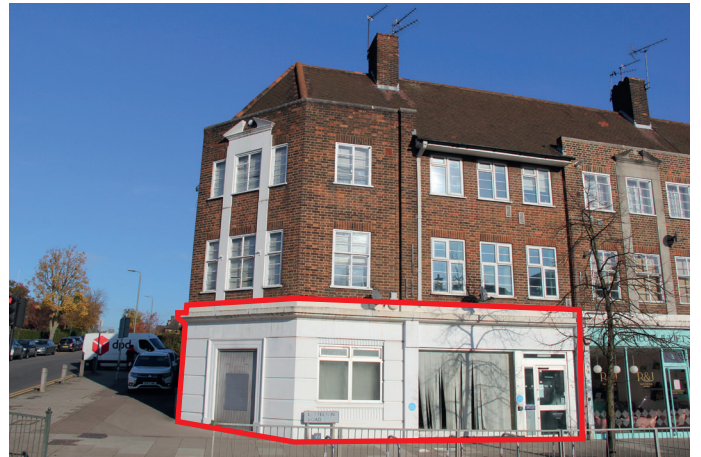
View of Rear Office Extension
