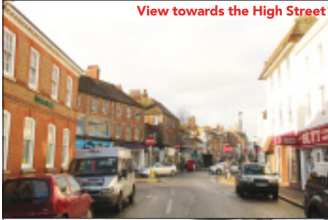
View towards the High Street
